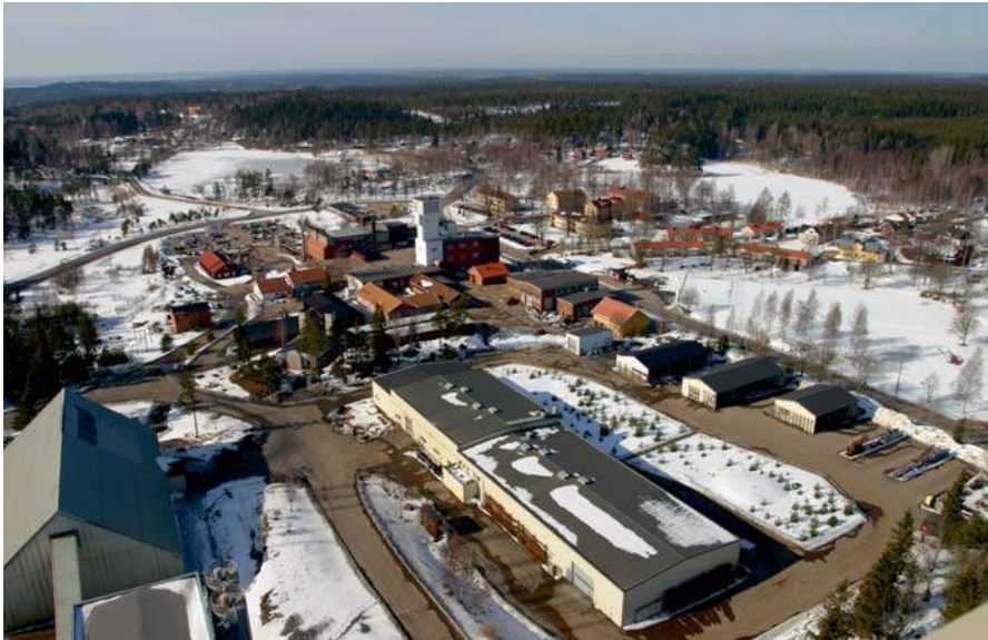
A view from the top of the ore treatment plant at Zinkgruvan. The mine has been in continuous production since 1857. The present day mill was constructed in 1976 and underwent a major modernization program during the early 1990s.
