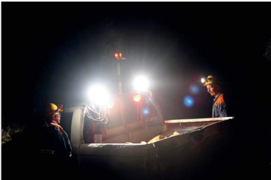
Work in progress at the Storliden Mine.
