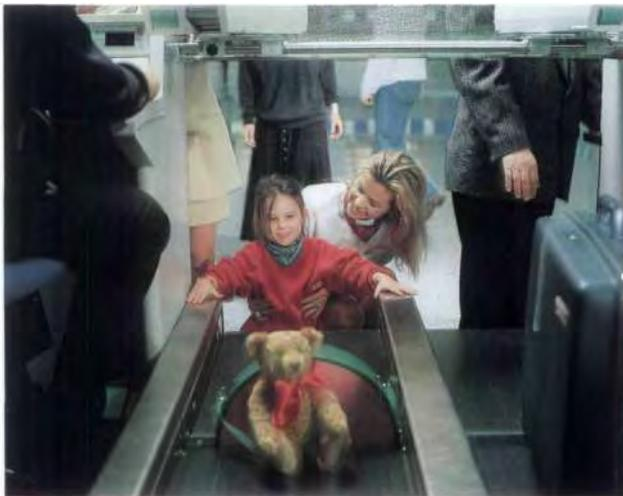
The fully automated, computer-controlled baggage conveyor at the Frankfurt airport transports luggage to its destination at a speed of 2.5 m per second.
