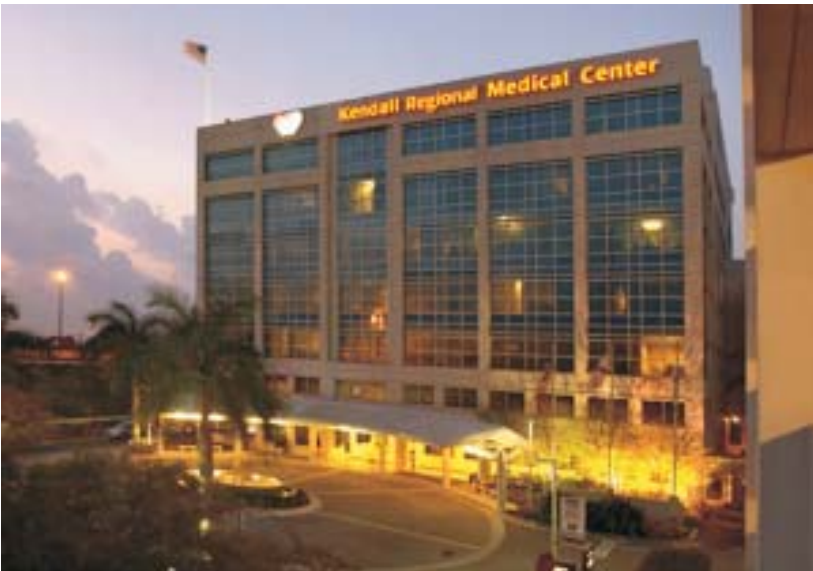
The Atrium Medical Offices at Kendall Regional Medical Center Miami, Florida 125,100 Rentable Sq. Ft.
