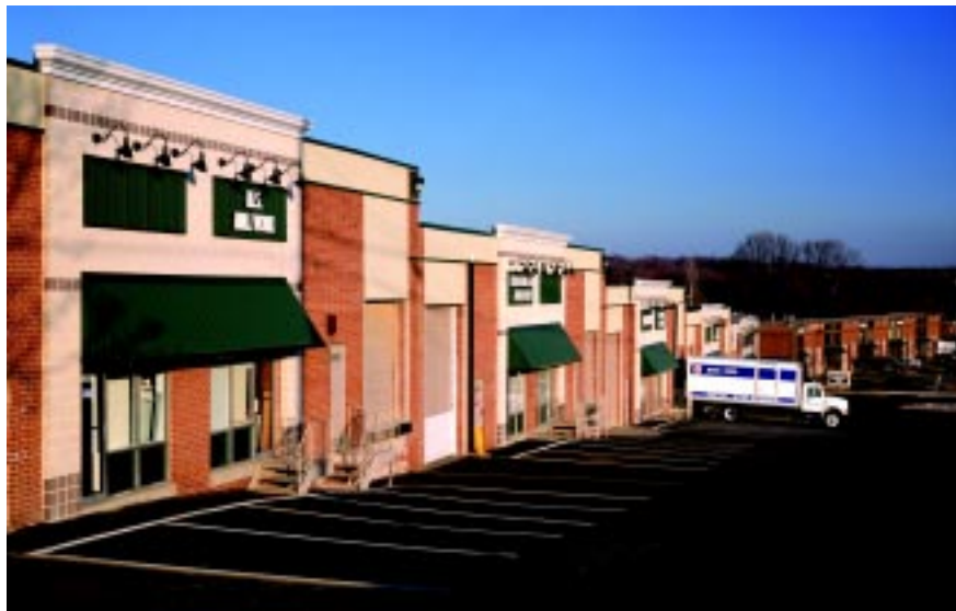
NVIP After Renovation
